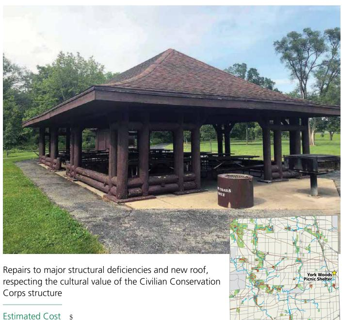
The project will correct several structural deficiencies. The log post and lateral post construction points of termination are failing, and the roof needs to be replaced. Substructure improvements also need to be addressed. Because the structure has a high cultural value, staff will develop a thorough reconstruction plan.
