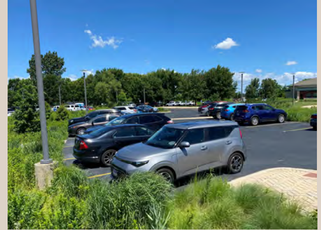
Parking Lot Improvements
