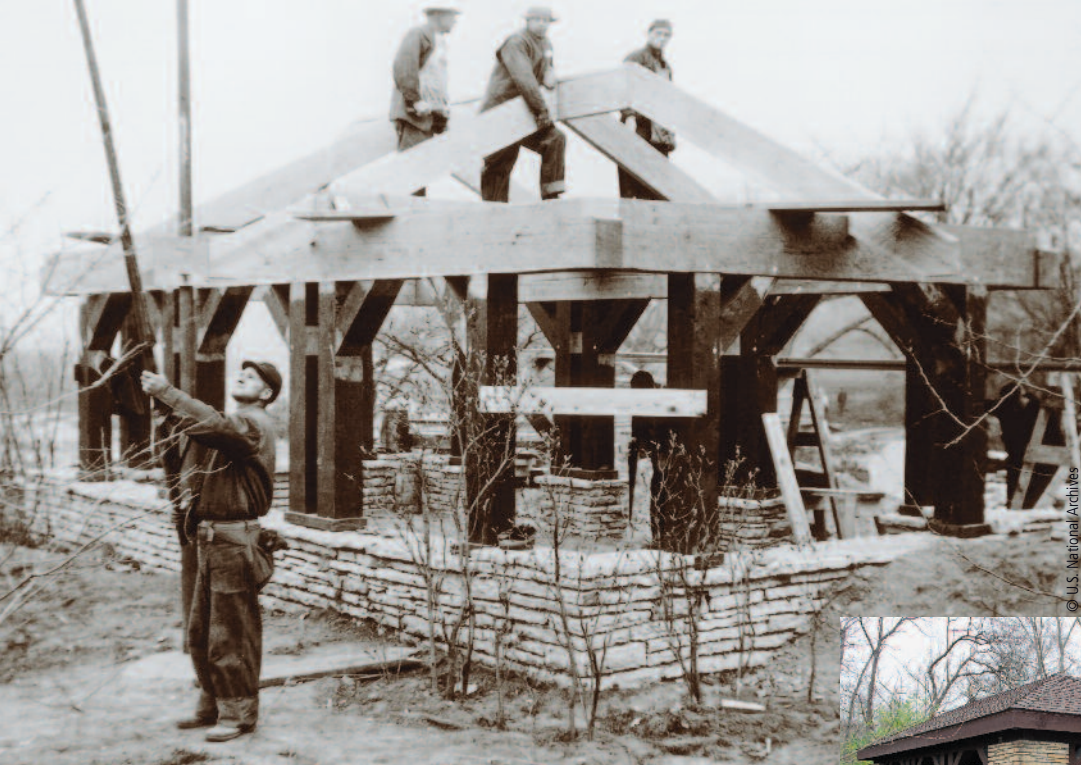
▲ The men of Camp McDowell frame the picnic shelter at Pioneer Park Forest Preserve and position a concrete arch for the footbridge over the West Branch of the DuPage River (top, left and center). Both structures welcome visitors today (bottom, left and center).
