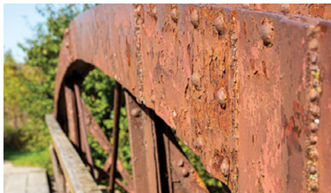
▲ Work on the 1870s bridge will refurbish the bridge's original wrought iron.
