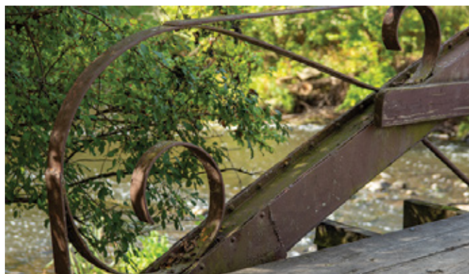
▲ The decorative railings keep people from walking over the arched top chord, which bends down to meet the wooden decking near each end of the bridge.
